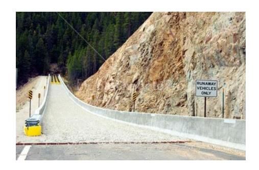
The gravel increases the time to impact, which decreases the impact force when the truck hits the barrels of water at the end.
